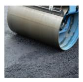
The intent of asphalt release agents is to eliminate harmful stripping products that come into contact with bituminous products and strip the asphalt (binding agent) from the aggregates causing potholes, ravelling, and other detrimental pavement failures.
